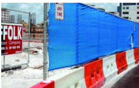
Temporary Construction Yards & Building Projects
