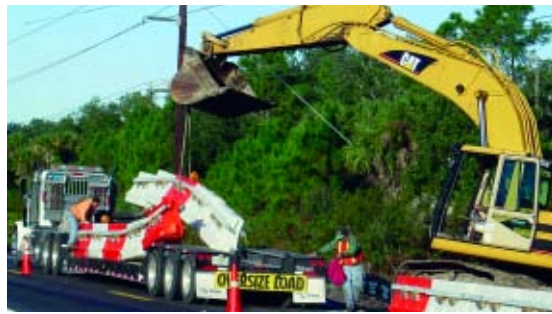
Transport & relocate assembled
