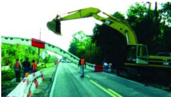
Relocation of 60 foot section
